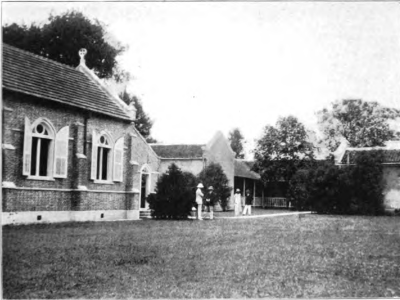
LEPER HOSPITAL, SIAOKAN Chapel and wards. This shows the possibility of orderliness in China
